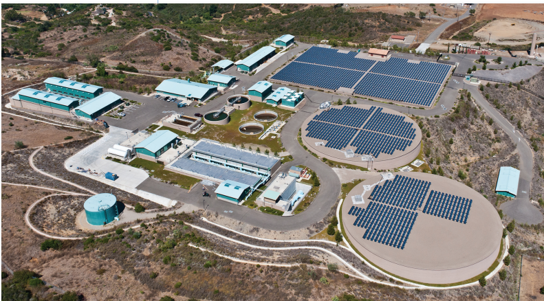
The 2003 master plan identified a need for additional water treatment for the region. The Twin Oaks Valley Water Treatment Plant was completed in 2008.
