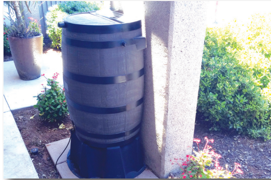
Rain barrels installed near the entrance to the Water Authority's headquarters distribute water through drip lines.
