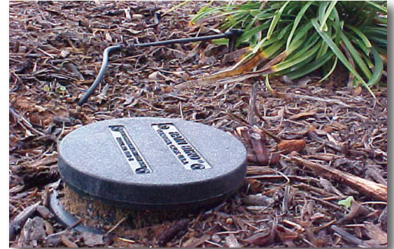
The water-efficient drip irrigation system around trees, shrubs and flowers delivers water to roots efficiently.
