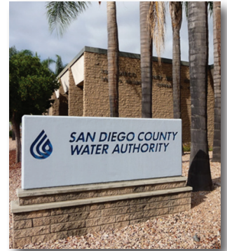
Landscaping rock reduced outdoor water use at the Escondido operations center.
