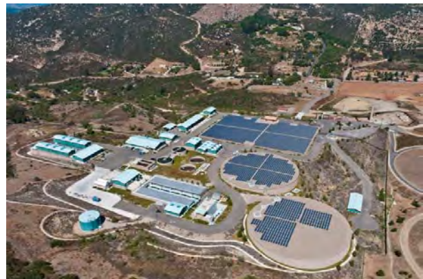
The 2003 Master Plan identified a need for additional water treatment for the region; the Twin Oaks Valley Water Treatment Plant was completed in 2008
