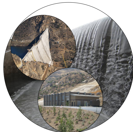
Optimization of existing facilities, like San Vicente Reservoir and Pump Station, to meet future demands will allow the Water Authority to provide improved reliability without additional capital investments.
