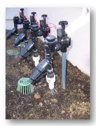
Low flow zone kit – valve, filter and pressure regulator
