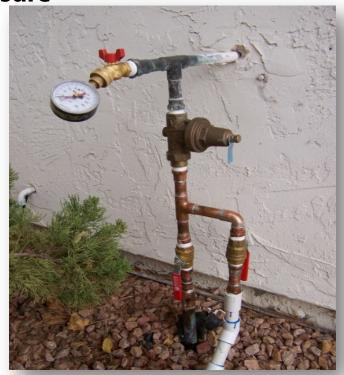
Static pressure at the point of connection (POC)- this may not always be a reliable location to measure irrigation pressure
