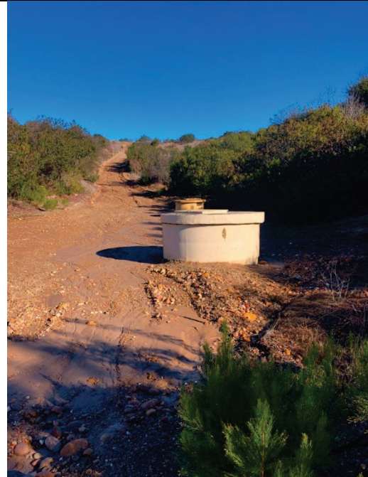
Photo 43 – (facing north) – Looking up the existing dirt access road at the erosion occurring along the road creating an erosional swale.
