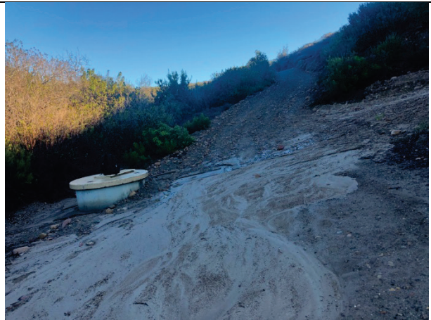
Photo 50 – (facing southeast) – Looking at the existing access road that is eroding adjacent to the unnamed ephemeral drainage 4.
