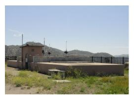
assessment identified seismic deficiencies and high relative risk for the Twin Oaks Diversion Weir Structure and recommended near-term rehabilitation. The 2021 study further developed high-level planning for improvements in the Second Aqueduct Diversion complex area including replacement of the Twin Oaks Diversion Weir Structure. The scope of this project currently includes the design and construction of a replacement for the Twin Oaks Diversion Weir Structure.
