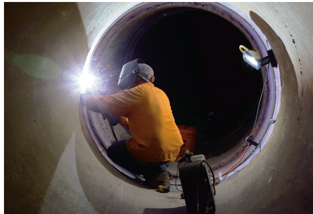
The Water Authority's Asset Management Program develops and uses innovative tools to maintain the region's 310 miles of large-diameter pipelines. The agency also aggressively relines and rehabilitates aging structures to ensure supply reliability.
