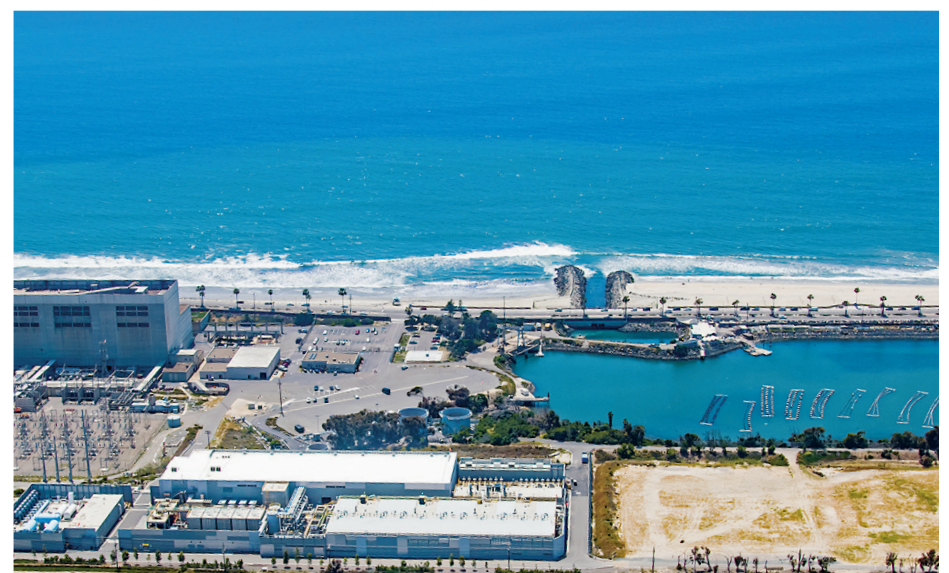
The Carlsbad seawater desalination plant sits next to Agua Hedionda Lagoon.
