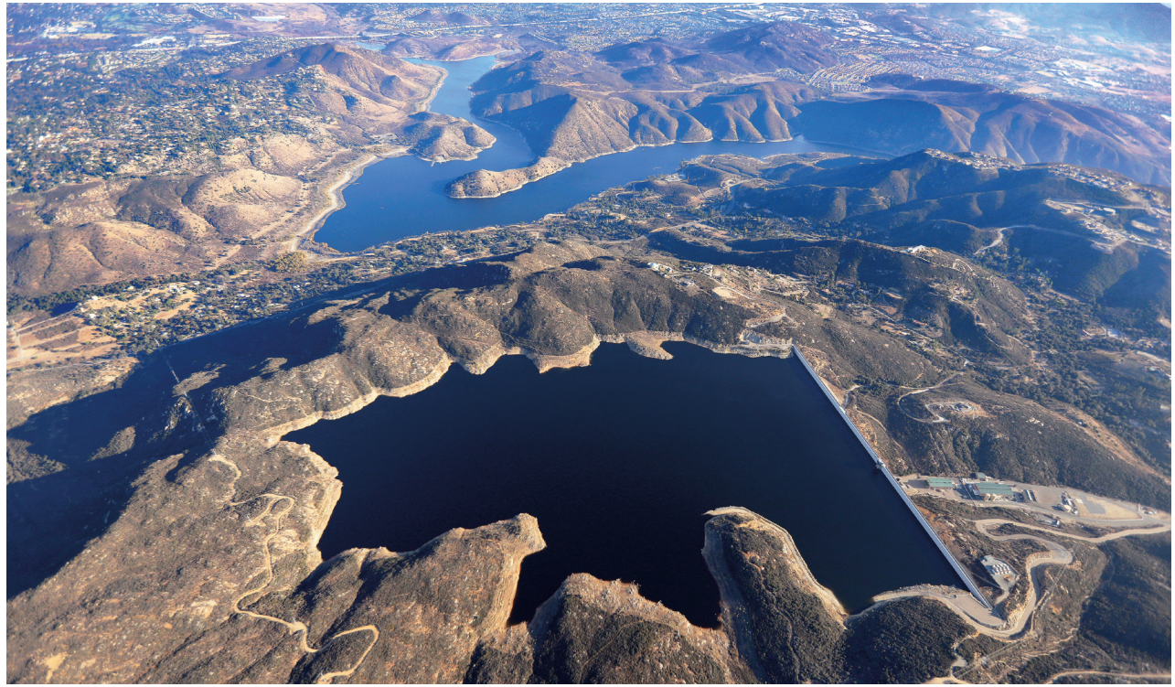
Completed in 2003, Olivenhain Dam is a major component of the Water Authority's Emergency & Carryover Storage Project, which protects the region in case imported water deliveries are interrupted, for instance, by an earthquake. Lake Hodges is in the background.
